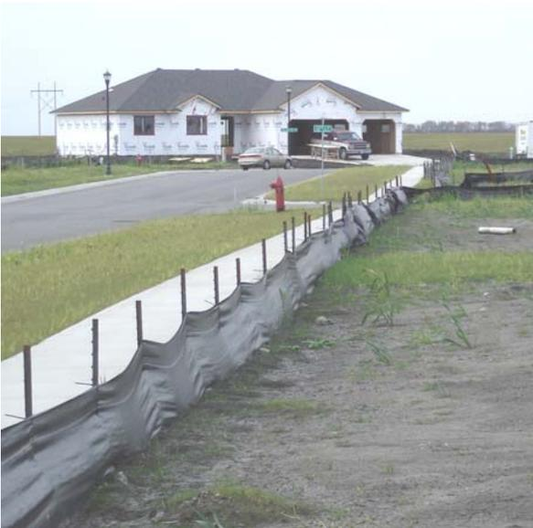
Typical silt fence installation with a grass buffer strip separating construction from final stabilization. Erosion has been minimized.
